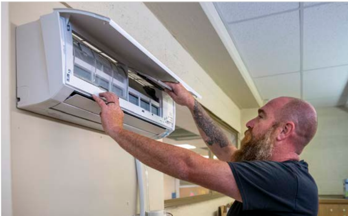
Lyon Mechanical installer Collin Schaale installs filters in a wall-mount unit.
