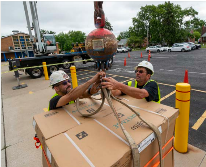
(left to right) Lyon Mechanical's Bob Fitzgerald and Ray Short rig condensing units to be craned to the roof of the school.
