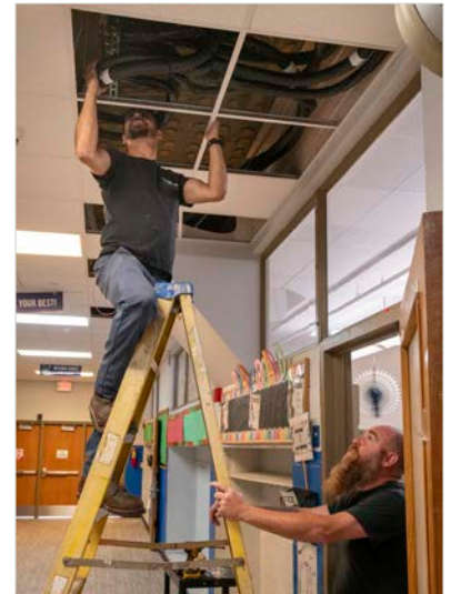
Lyon Mechanical installers Bob Fitzgerald and Collin Schaale run linesets.
